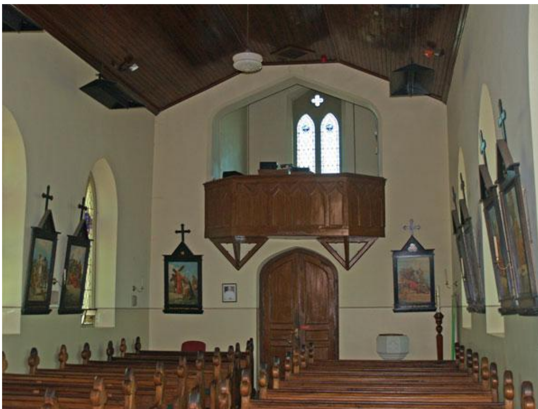
Thomas' tower gallery with Goodridge's original nave west door beneath it (Image: Brian Andrews)
