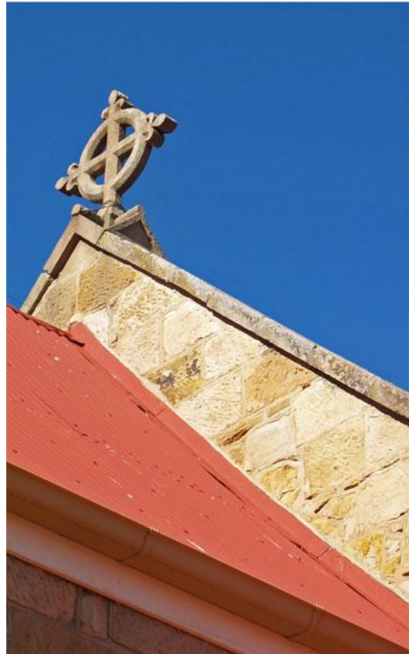
At left, the chancel east gable cross, copied from a stone exemplar; at right, the nave east gable cross, also copied from exemplar stonework. Note the steeper slope of the chancel roof, a compromise by Thomas between the chancel roof slope on Pugin's model and the shallow pitch of Goodridge's Gothic nave roof (Images: Brian Andrews)
