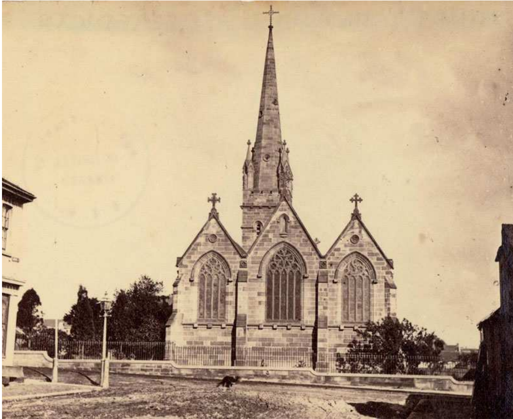
Liturgical east elevation viewed across George Street West, last quarter nineteenth century (Courtesy: Mitchell Library, State Library of New South Wales)
